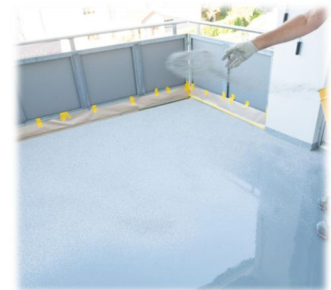
Anti slip epoxy floor
